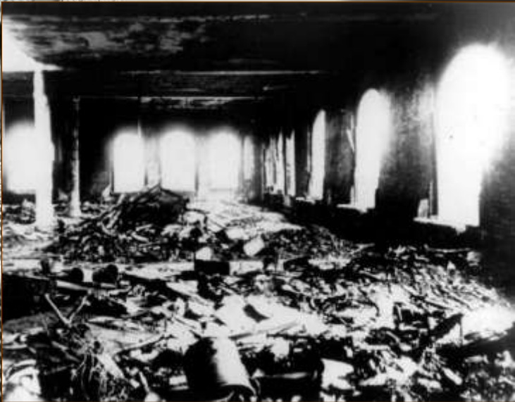
10 th Floor After the Fire
