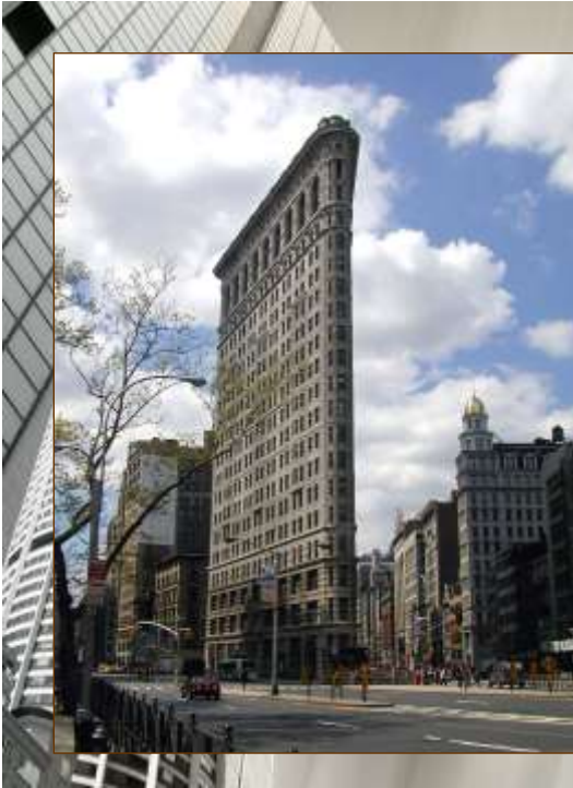
Flatiron Building NYC – 1902 D. H. Burnham
